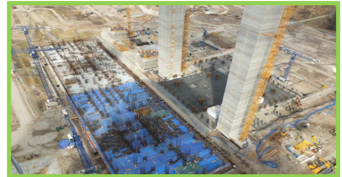
Use of slag cement for basements and massive construction parts for a power plant in Poland
